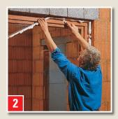
Cut off excessive material with a sharp knife after about 2 hours.
