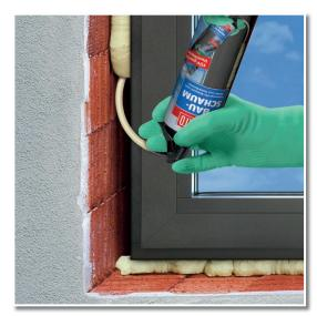
Filling a connection joint on the window.
