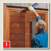
Foaming a window frame: Shake the BAUSCHAUM can well about 20 times. Foam around the window frame.
