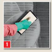
Stir bag contents (5 kg) in approx. 1.4L of clean water. Stir again after 5 minutes. Slurry the grouts with a sponge rubber board diagonally into the joints. Skim off excess material.
