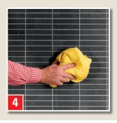
Polish the tile flooring with a dry cloth as soon as the mortar has hardened.
