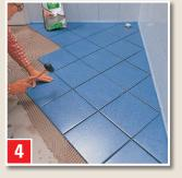
Bonding tiles to a heated screed on the floor: Knock on the tiles with a rubber mallet. Grout on the floor after 2 days, on the wall after 1 day.
