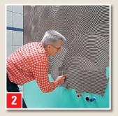
Bonding tiles in a shower: SICHERHEITSKLEBER Apply FLEXIBEL to DUSCH-ABDICHTUNG and comb it with a toothed trowel
