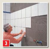
Tiles can be inserted and aligned within 30 minutes.
