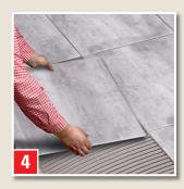
"Scratch" the adhesive thinly onto the substrate as a contact layer. Directly thereafter, apply a thicker layer immediately and comb through to the substrate with a toothed trowel. Pull the toothed trowel over the surface at an even angle between 45–60°.
