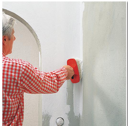
Brightens up the substrate and gives the wall grip for textured plaster.
