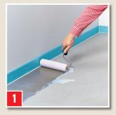
Apply BESTE BASIS on the substrate with a paint roller and allow drying for 1 to 4 hours depending on the absorbing capacity.
