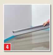
The required system covering of 5 mm is measured by dipping an aluminium straight edge and measuring the adhering mortar film. Immediately clean the tool with water
