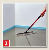
Evenly spread the applied mass with a scraper or a rubber slider. Protect the fresh material from draught and sunlight.
