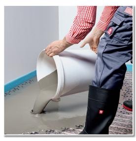
Self-spreading and creates level surfaces on e.g., thin-layered floor warming systems.
