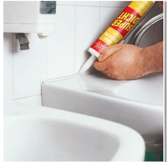
Sealing the joint at the washbasin permanently elastic.
