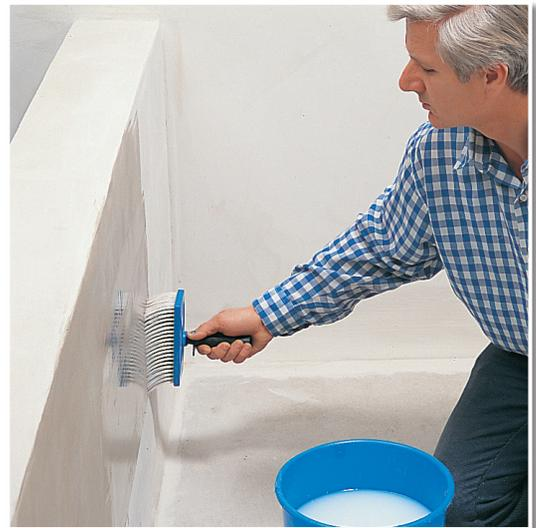
Primes an absorbent plaster before subsequent work, e. g., painting.
