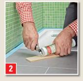
Cut off the nozzle tip at an angle (according to the joint width) and the tip of the cartridge.
