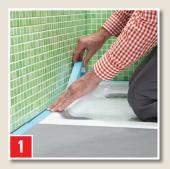
Before beginning the flexible sealing, tape the joint edges with masking tape.
