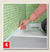
Smooth within 20 minutes using a moistened WIE GUMMI FUGENGLÄTTER (water with 10 % detergent additive). Immediately remove masking tape, re-smooth joint edges.
