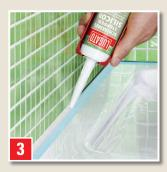
Squeeze SCHIMMEL-STOPPER-SILICON generously into the joint using the cartridge applicator gun.
