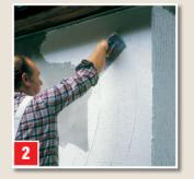
Stir the plaster with a stirrer. Apply a thin layer of ROLLPUTZ with a smoothing trowel (1-2 mm). Use rust-free tools.
