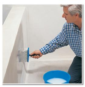
Primes an absorbent plaster before subsequent work, e.g., painting.
