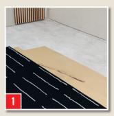
Apply AKUSTIK-PANEEL-KLEBER to the rear of the panels in vertical strips, approx. 9 mm wide and evenly spaced. (Colour of adhesive is black)
