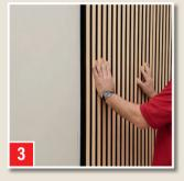
Align panels and press on firmly. With large, heavy panels, additional mechanical fixing is recommended.
