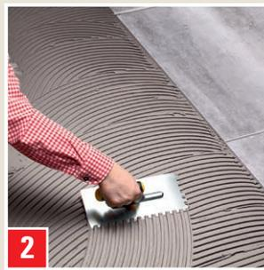
2 "Scratch" the adhesive thinly onto the substrate as a contact layer. Directly thereafter, apply a thicker layer immediately and comb through to the substrate with a toothed trowel. Pull the toothed trowel over the surface at an even angle between 45–60°.
