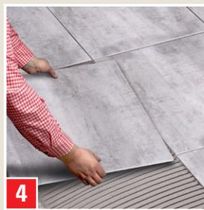
4 Insert, align and press the tiles within 30 minutes.
