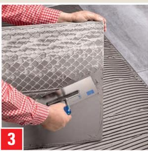
3 Outdoor tiles, under water; for highly stressed surfaces and tiles with an edge length of 50 cm or more, glue indoors with minimal cavitation. To do that, apply additional adhesive to the back of the tiles, approx. 2 mm thick.
