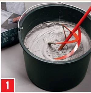
1 Stir the contents of the bag (20 kg) into 7.2–8 litres of clean water. Stir again after approx. 3 minutes.
