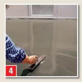
Support the meshes with a smoothing trowel, if necessary use a spiked roller or a garden rake. Protect fresh material from draughts and sun.
