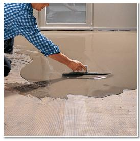
NEU AUF ALT! creates a level surface for paintwork and floor coverings.
