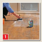
Spread the BESTE BASIS with a mop. Let dry for at least 4 hours. Attention: Do not forget the edge insulation strips!
