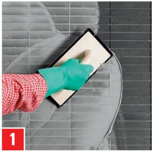
1 Stir bag contents (5 kg) in approx. 1.4L of clean water. Stir again after 5 minutes. Slurry the grouts with a sponge rubber board diagonally into the joints. Skim off excess material.
