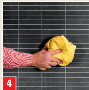
4 Polish the tile flooring with a dry cloth as soon as the mortar has hardened.
