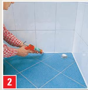
Provide the floor joint with a permanent elastic seal before placing the shower tub in place.
