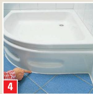
Smooth the sealant with a wet finger or the silicone smoothing tool FUGENGLÄTTER within 10 minutes (water with 10% colourless washing-up liquid).
