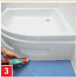
Seal the connection joint between the shower tub and floor tiles.
