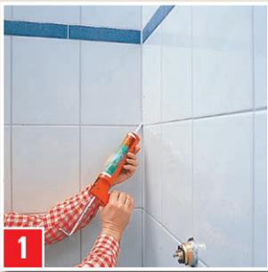
Provide the corner joint with a permanent elastic seal.
