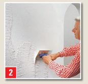
Stir the plaster with a stirrer. Place plaster onto a steel trowel and apply. Use rust-free tools.
