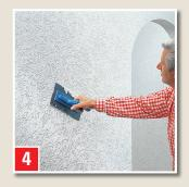
Create texture with a plastic smoothing tool within 10–20 minutes. Apply in a horizontal, vertical, circular or diagonal direction.
