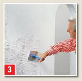
Apply and then skim to the grain thickness with a steeply angled steel trowel.
